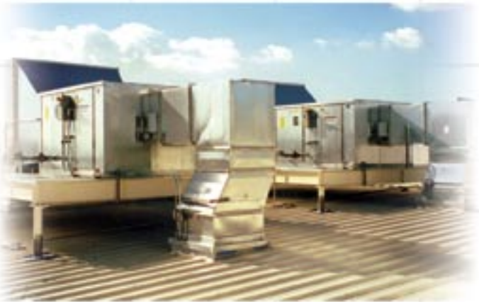
Air make-up units with temperature and humidity control for critical applications
